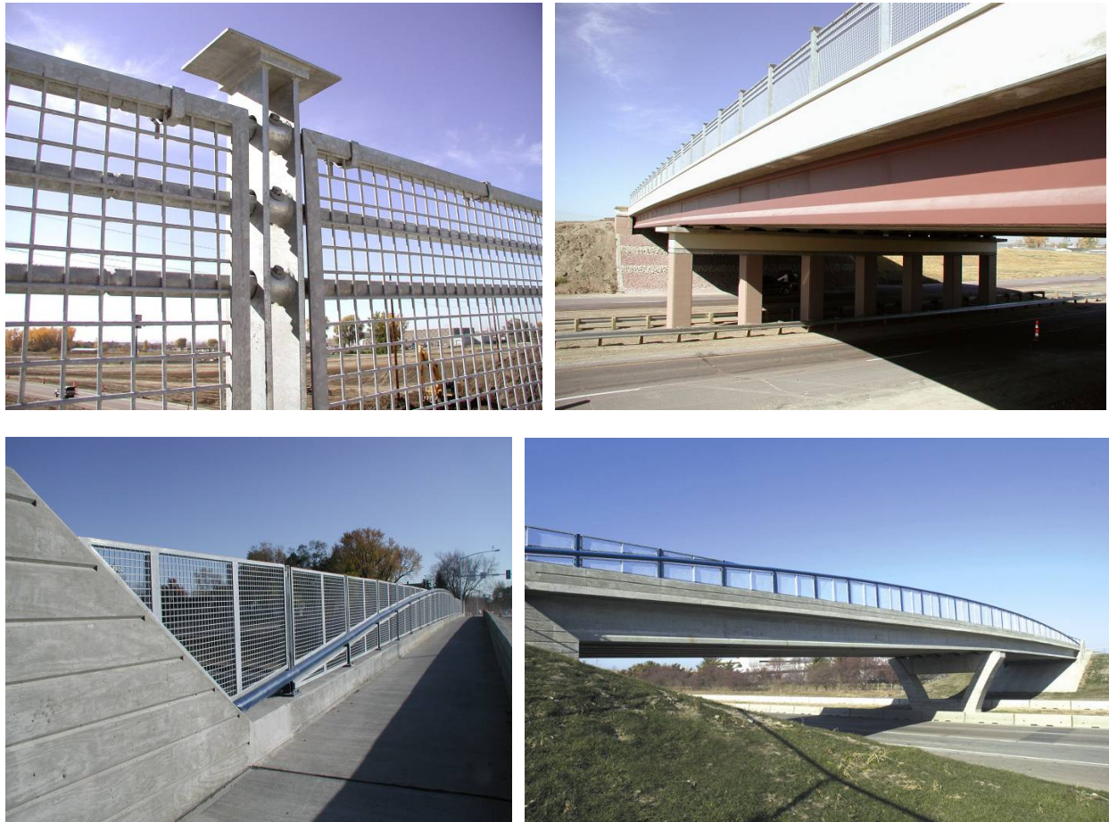
Figure 9.5.3.7-2. Bridges with complementary bolt-on aesthetic details
