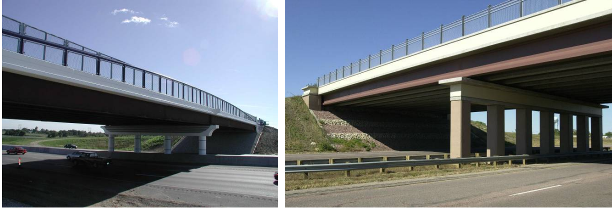
Figure 9.4.3. Level “B” bridge examples in Iowa
